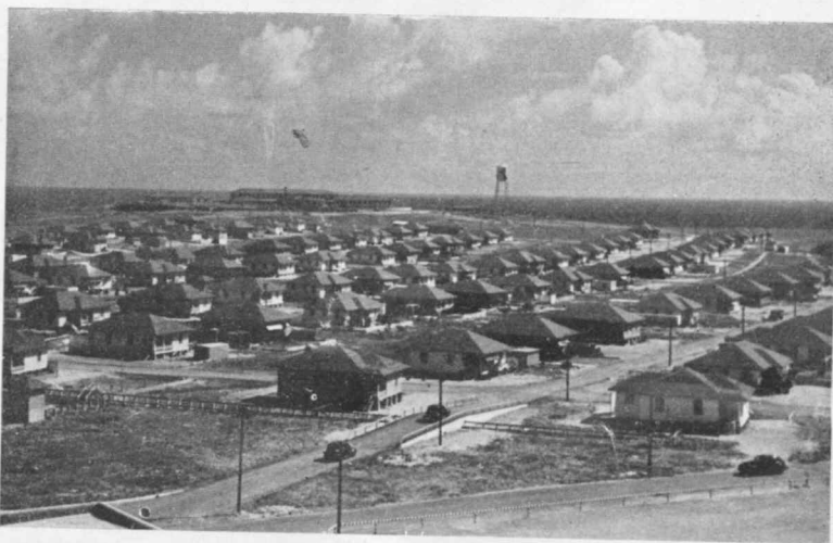
Shown above is a portion of the residential colony, which includes approximately 500 bungalows for employees who have their families at Aruba
