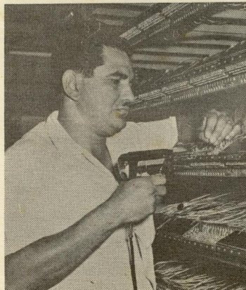
G. Arends makes crossconnection at Telephone Exchange for new personal numbering system.
