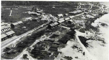
View east in 1928 from Powerhouse No. 1 area. 1. Present Cracking Plant area. 2. Site of "Cat Cracker." 3. Old Hospital, later Personnel Office, now site of "Cat Cracker" compressor houses. 4. Bungalows 1-15, now site of Laboratory, General Office, and Powerhouse No. 2. 5. Main refinery road, the only thing unchanged.
